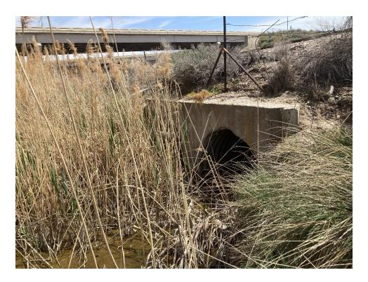
Photo 30: Looking upstream at CDWB25 4-ft CMP and 4.25-ft CMP culvert.
