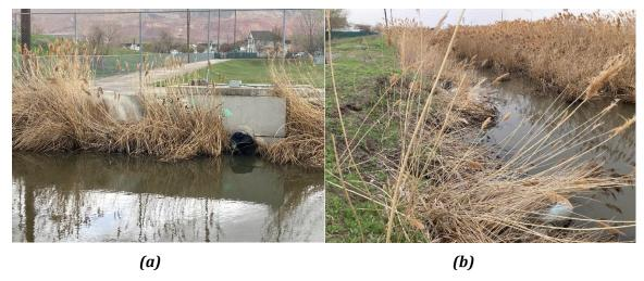
Photo 2-8: Storm Drain Pipes with (a) and without (b) back flow preventor
