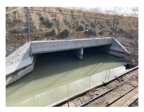
Photo 10: Standing on top of CDW5 bridge looking upstream at CDW6 I-215/Legacy Parkway double 13-ft x 7-ft culvert.
