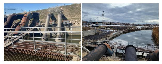
Photo 2-10: Evidence of Corrosion and Rust on Existing Lift Station
