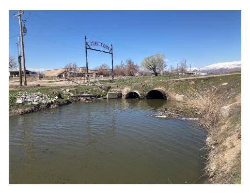
Photo 14: Looking downstream at CDWB10 5-ft CMP and 6-ft CMP culvert.
