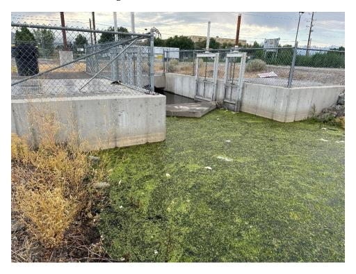
Photo 21: Looking downstream at CDWB17 2200 West double 4-ft RCP culvert.
