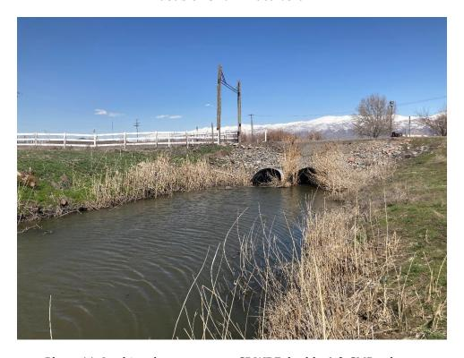
Photo 11: Looking downstream at CDWB7 double 6-ft CMP culvert.
