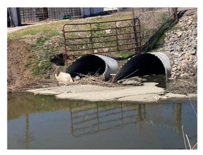
Photo 2-3: Example of Collapsed Culvert at 2441 North Rose Park Ln.
