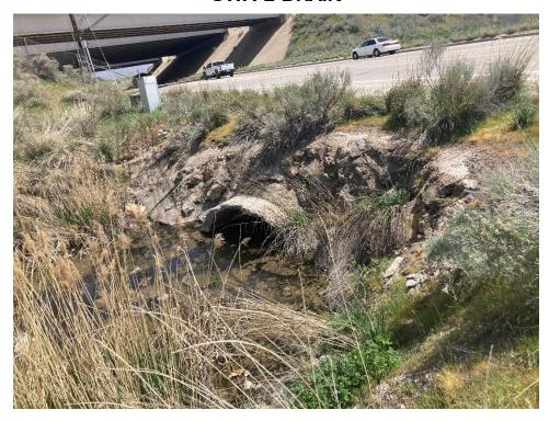
Photo 31: Looking upstream at CWA2D1 500 South 7-ft RCP culvert.
