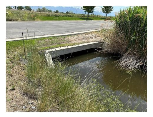
Photo 20: Looking downstream at CDWB16 13-ft x 4-ft culvert.
