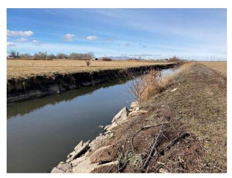
Photo 6-1: Example of Concrete Debris on Right Bank of Sewage Canal
