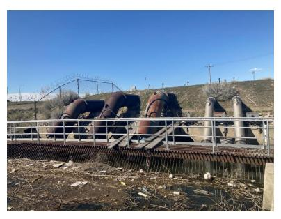
Photo 2-1: Existing Lift Station Pumps
