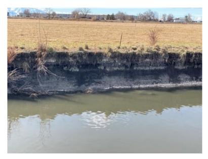
Photo 2-7: Vertical Banks on the Sewage Canal with Sediment Deposited at Toe of Bank
