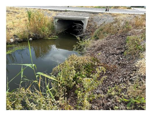
Photo 22: Looking downstream at CDWB18 2360 West 8-ft x 5-ft culvert.
