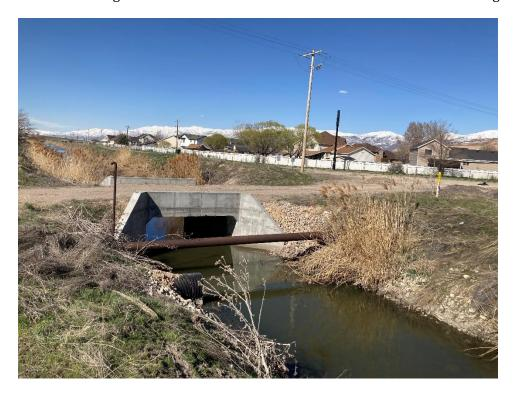
Photo 17: Looking downstream at CDWB13 1800 North 11-ft x 5-ft box culvert.
