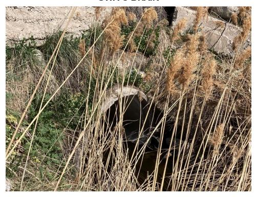
Photo 33: Looking downstream at CWA3D2 5-ft RCP culvert.
