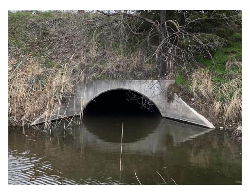
Photo 24: Looking upstream at CDWB21 North Temple 9-ft CMP culvert.
